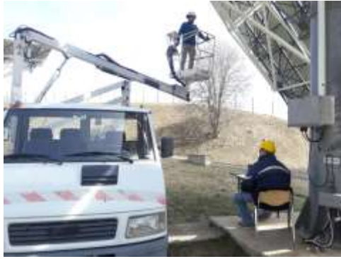
Figure 2. Adjustment of a heliostat's mirrors using a bucket truck
