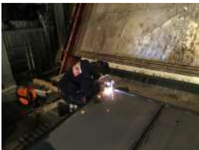
Welding of the metallic protection
