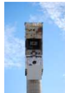
View of the Next-CSP aperture with metallic protection
