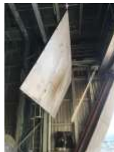
Metallic protection lifted and installed to block the concentrated radiation
